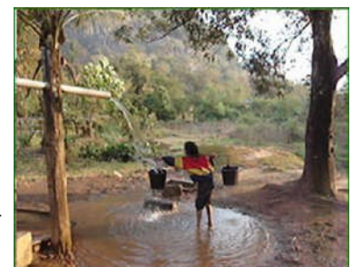
A villager uses the new gravity fed water system in Kaengyalouan Village
