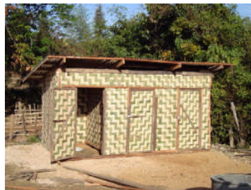
Latrine block in Phonkham village
