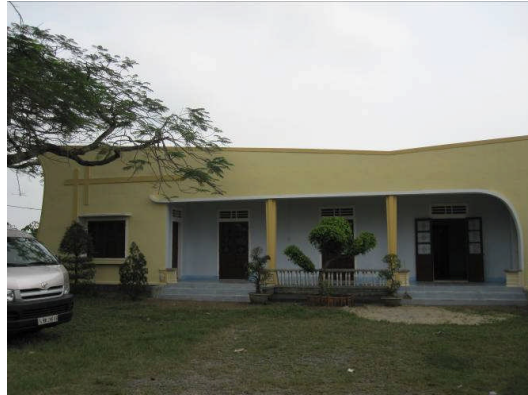
Exterior after repairs
