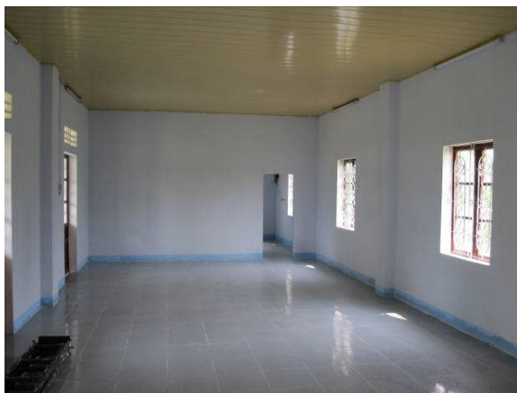
Interior after repairs
