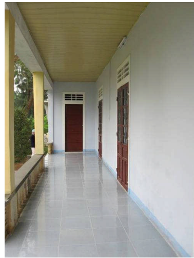
Walkway after repairs
