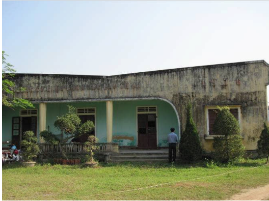
Exterior before repairs
