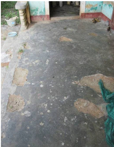
Walkway before repairs
