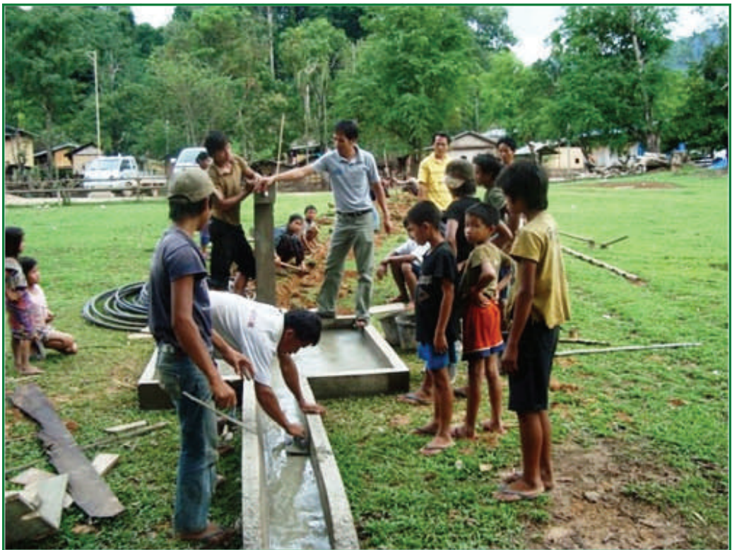
Completing the construction of the water pump in the school ground for the gravity-fed water system in Thongkong Village
